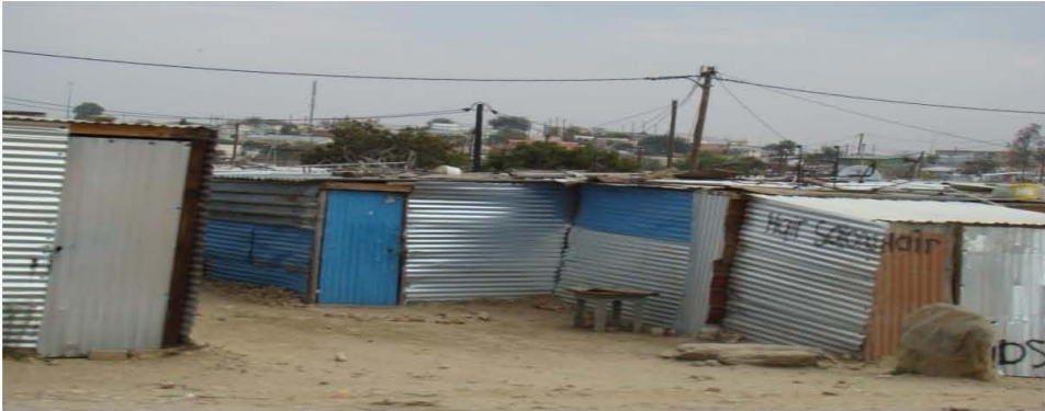
Figure 3.4: Low, Middle and High-Income Housing in Windhoek
